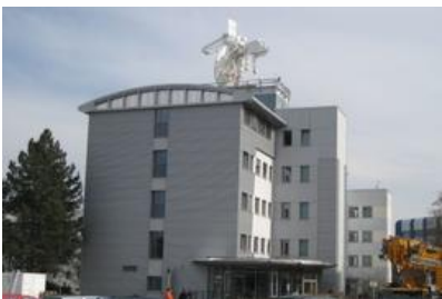
Radarantenna on top of the Institute Building
